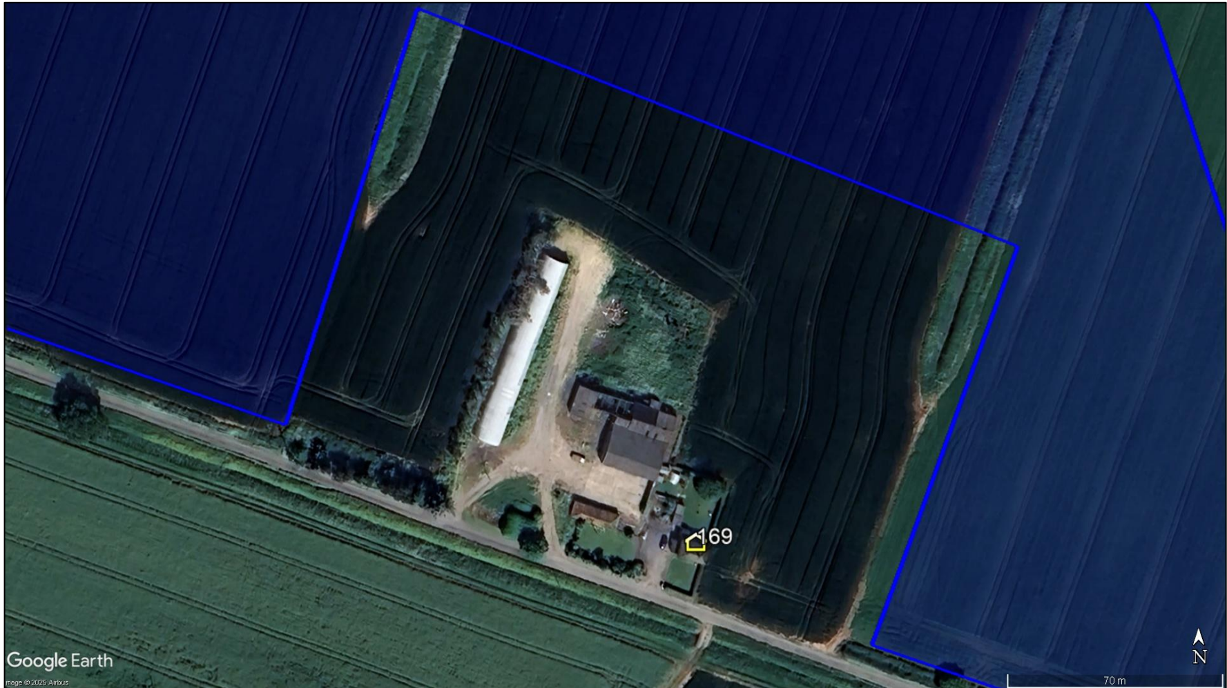
Dwelling receptor 169 – aerial image
