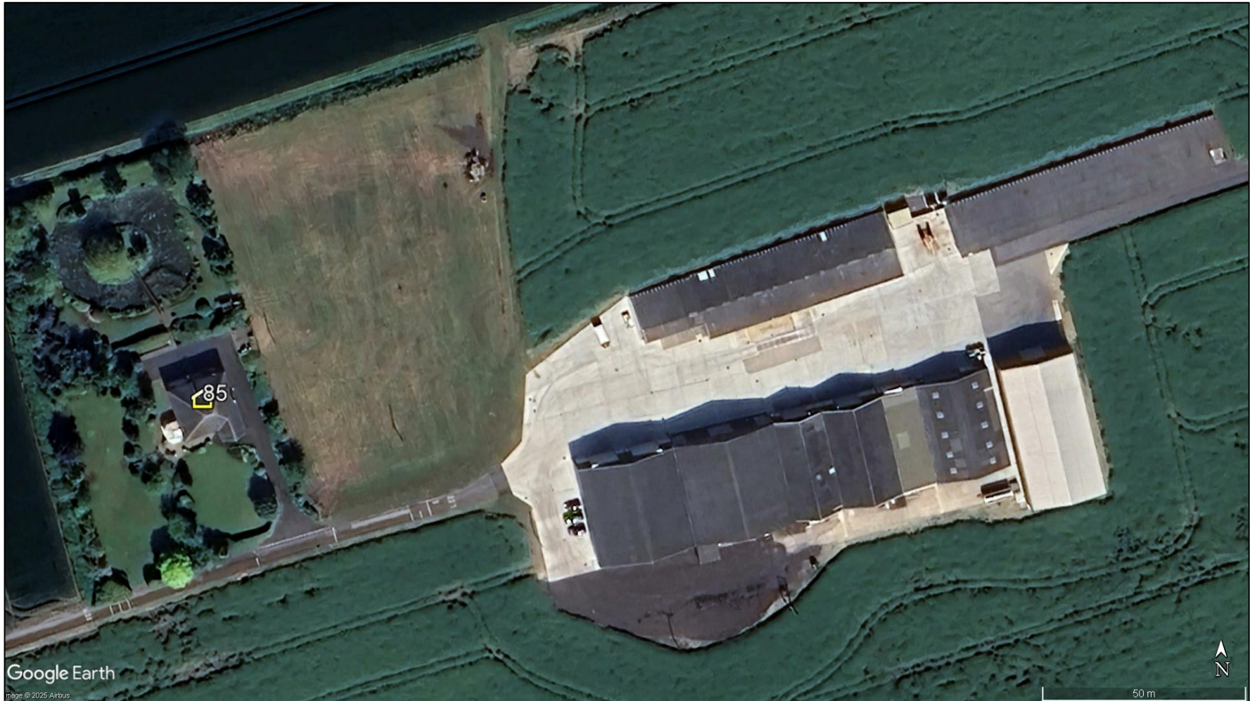
Dwelling receptor 85 – aerial image
